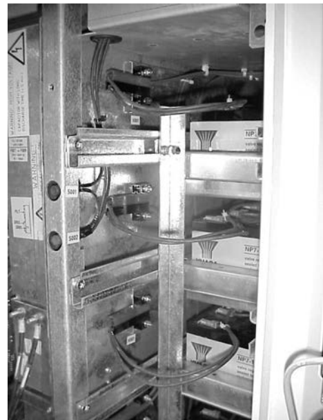
Connect all battery drawers to the terminal on the left side of the column
