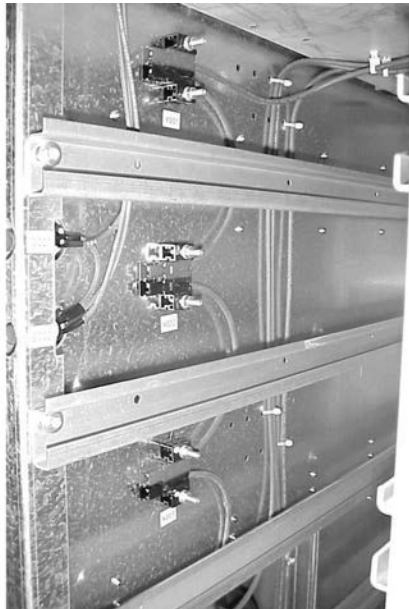
Insert battery drawers in the APC Silcon UPS
