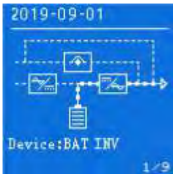
Figure4-5 Battery Inverter Output
