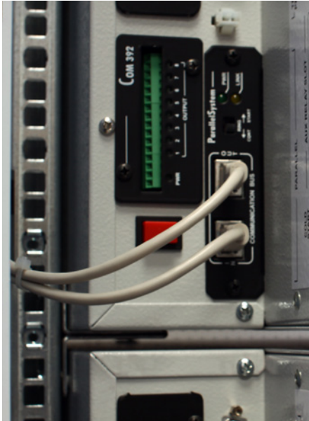
Parallel configuration and programmable relay contacts board.
